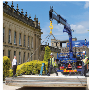
Delivered and installed utilising our fleet of specialist vehicles and fully accredited installation teams
