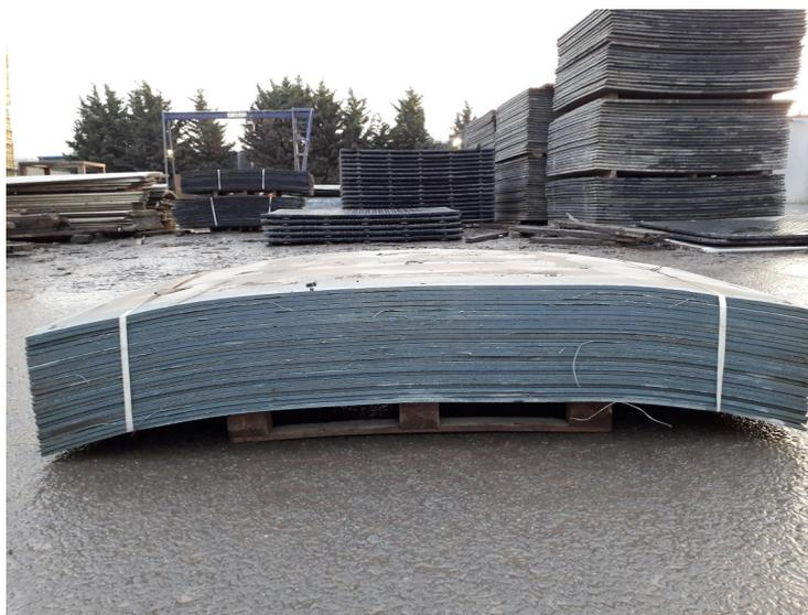
LD mats will be delivered stacked 25 per pallet and banded. Position the stack in a clear, level area in close proximity to the planned installation.
