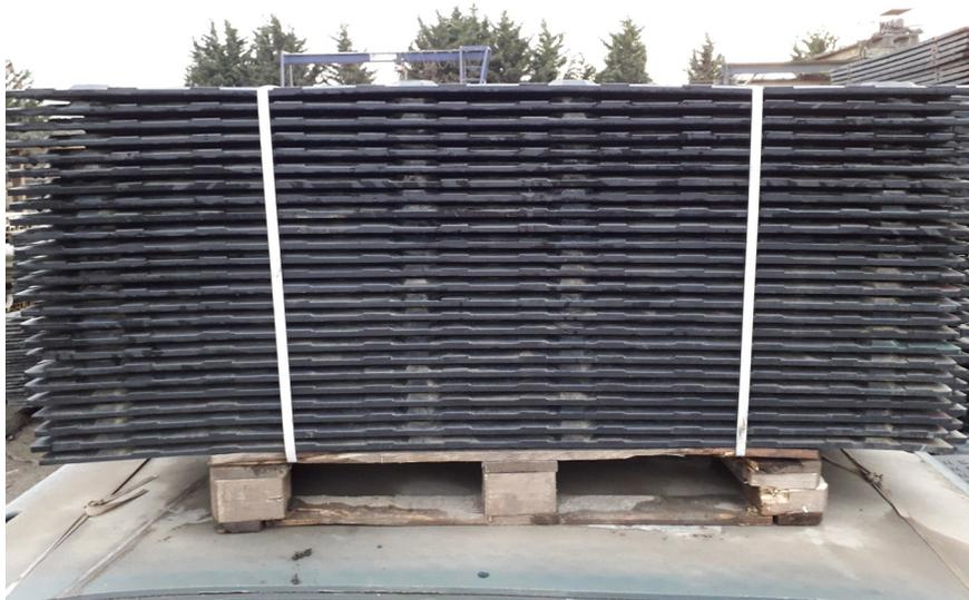
MaxiTrack mats will be delivered stacked 25 per pallet and banded. Position the stack in a clear, level area in close proximity to the planned installation.
