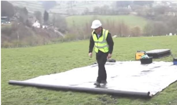
1. If required, install a geo textile membrane: this is usually used on longer duration projects.
