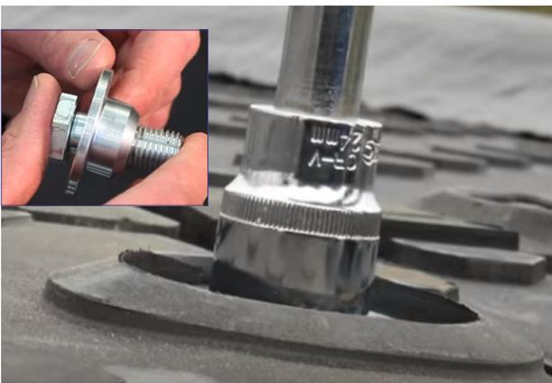
3. Self-aligning collars and low profile bolts are used to connect the mats (see inset top left). Use a 24mm socket to tighten the bolts.
